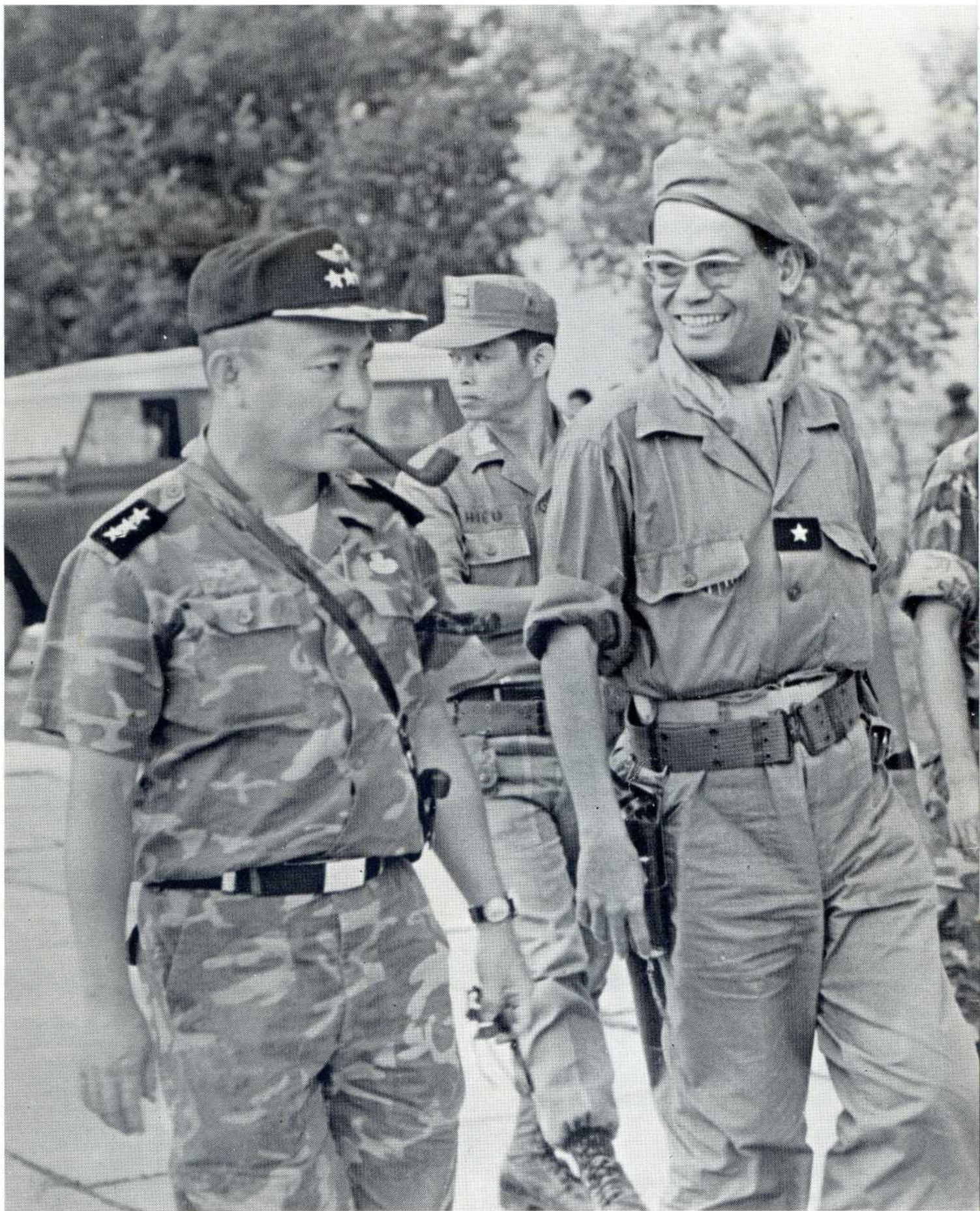
Lieutenant General Do Cao Tri (left) and Mr. So Phiek Phoeck, Minister of Public Works for the Government of Cambodia inspect a bridge recently rebuilt by the ARVN 303rd Combat Engineer Battalion near Svay Rieng.
